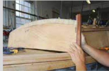
The cabin front is then manoeuvred into place and trimmed to fit. Note the curve top and bottom, which will be filleted into place.
