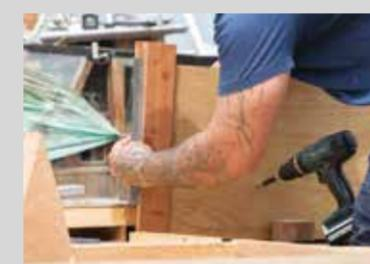
**2** Jesse checks the measurements with a steel ruler, ideal as it gives a straight edge that resists being warped, unlike a flexible steel tape.
