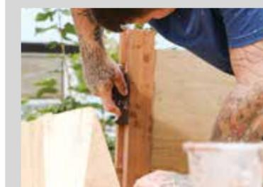
**3** Any adjustments are made with a small hand plane or sharp chisel. With all tools, the sharper the blade the better the results.
