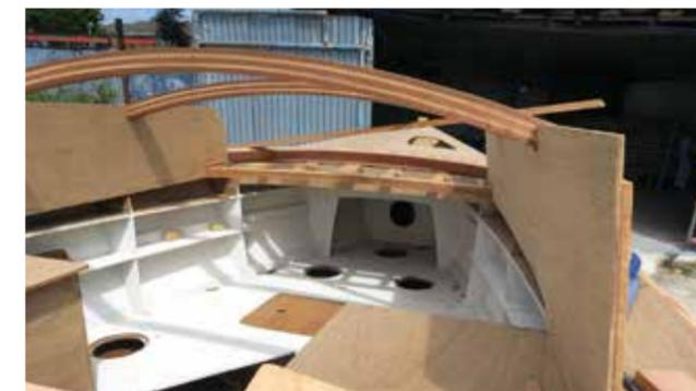
The forward shelf at the front of the cabin came in at a different width than expected, so the team have been working to compensate for the irregularity
