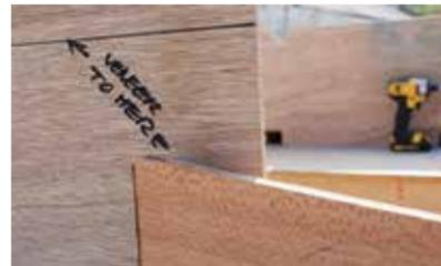
The coaming curves in to meet the cabin sides, with various options for making the join a decorative one
