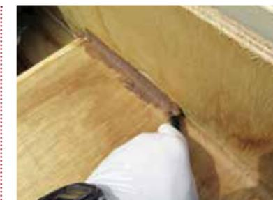
Filleting involves running a bead of thickened epoxy along the join line between two pieces of timber. West System 405 Filletting Blend gives the epoxy its brown colour and assists in creating a strong bond
