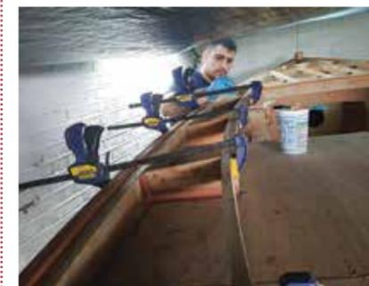
LEFT Boatbuilder Jesse Doyle secures the detached timber with adjustable clamps to pull the two pieces together. RIGHT A mix of thickened West System epoxy is then applied in fillets along each join
