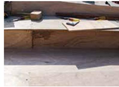
The beams are then covered with 12mm plywood. Once filleted into place, the cockpit sole will be self-draining
