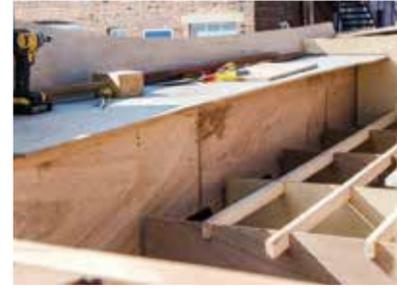
The support the weight of potentially four big sailors, the frames under the cockpit floor support several longitudinal beams
